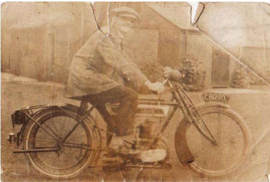
CB1280 is much easier to identify as a Levis flat-tank two stroke.
